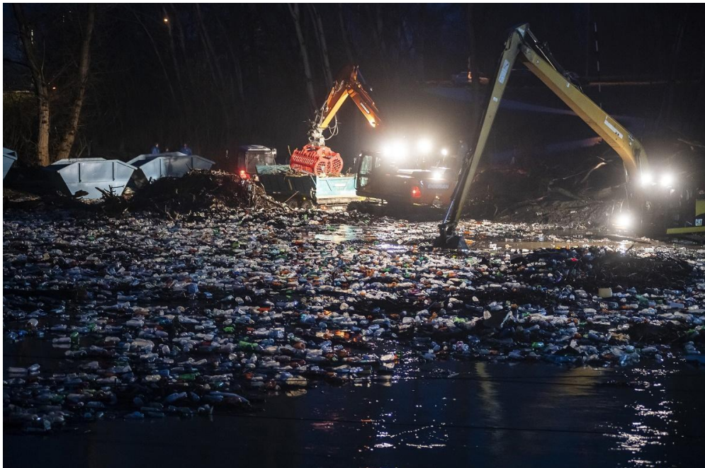
Massive riverine waste pollution – the so-called plastic flood – is under elimination at the Upper Tisza Photo: FETIVIZIG
