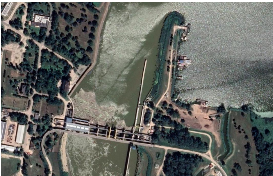
Accumulated waste visible from the air at Kisköre HPP. Source: Google Earth
